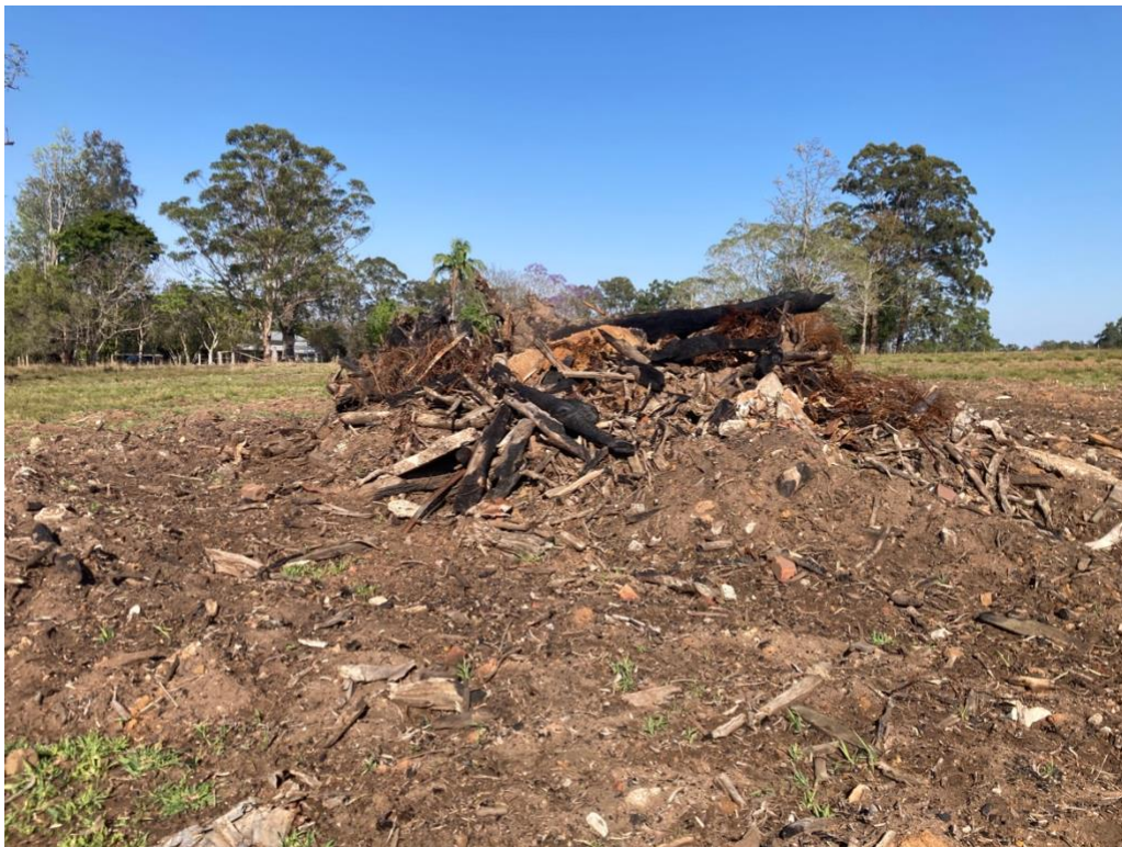
Burn pile of materials from recent demolition of structures
